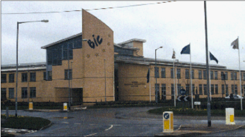
Positive steps for North London and the Lee Valley - The Business Innovation Centre, Innova Park
